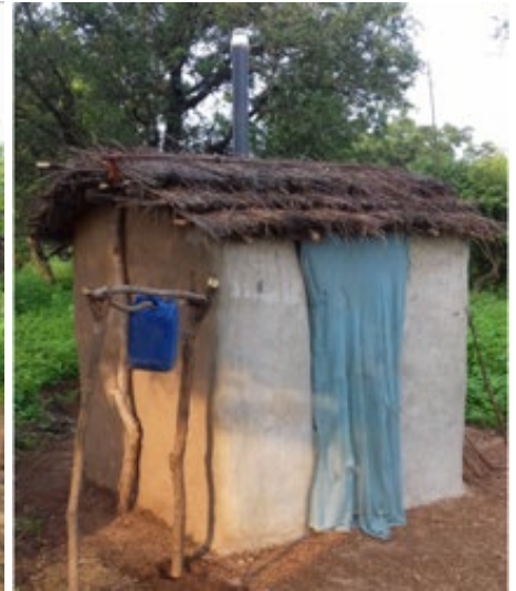
Toilet with net as door
