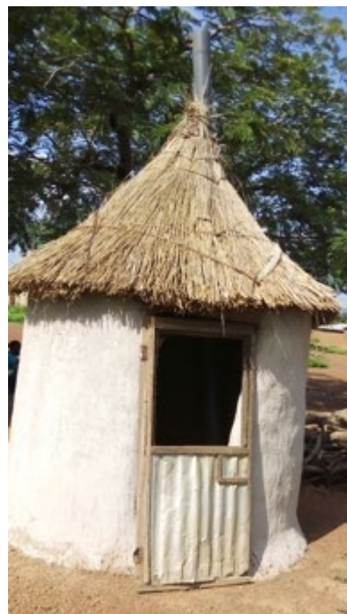
Toilets with round walls made of mud + cow dung plastering
