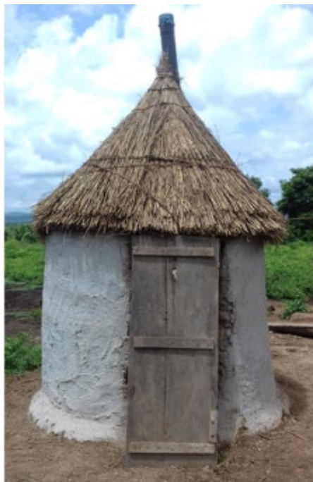
Toilets with round walls made of mud + cow dung plastering
